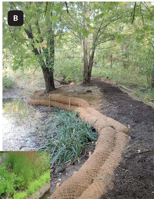
FIGURE 4.10 EXAMPLES OF TYPES OF ACCESS POINTS Real-life examples of the variety of access points recommended for implementation at Chandler Pond. A - Boulder-Reinforced B - Log/Coir Log-Reinforced C - Raised Platform
