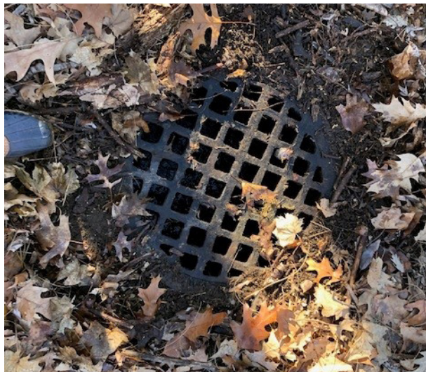
FIGURE 2.10 AREA DRAIN IN THE WOODLAND AREA This area drain connects to inlet pipe B, draining into the pond.
